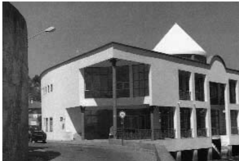
Figure 3.13 Bus Station, Tavira, Portugal
