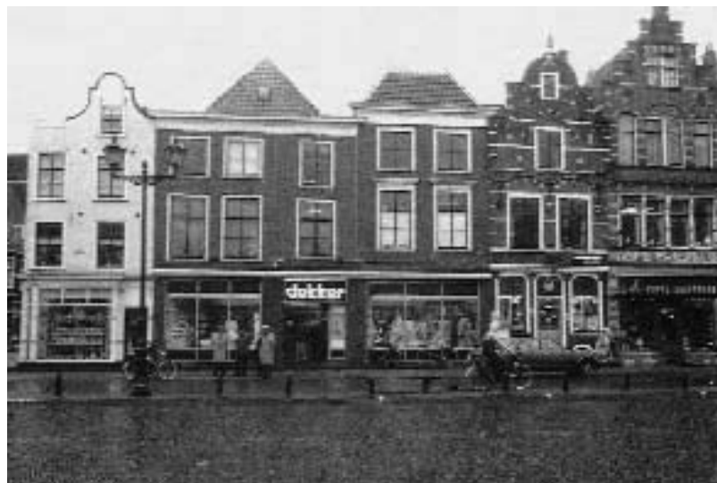
Figure 5.15 Paved square, Delft
