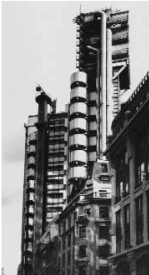
Figure 4.12 Lloyds Building, London, designed by Richard Rogers
